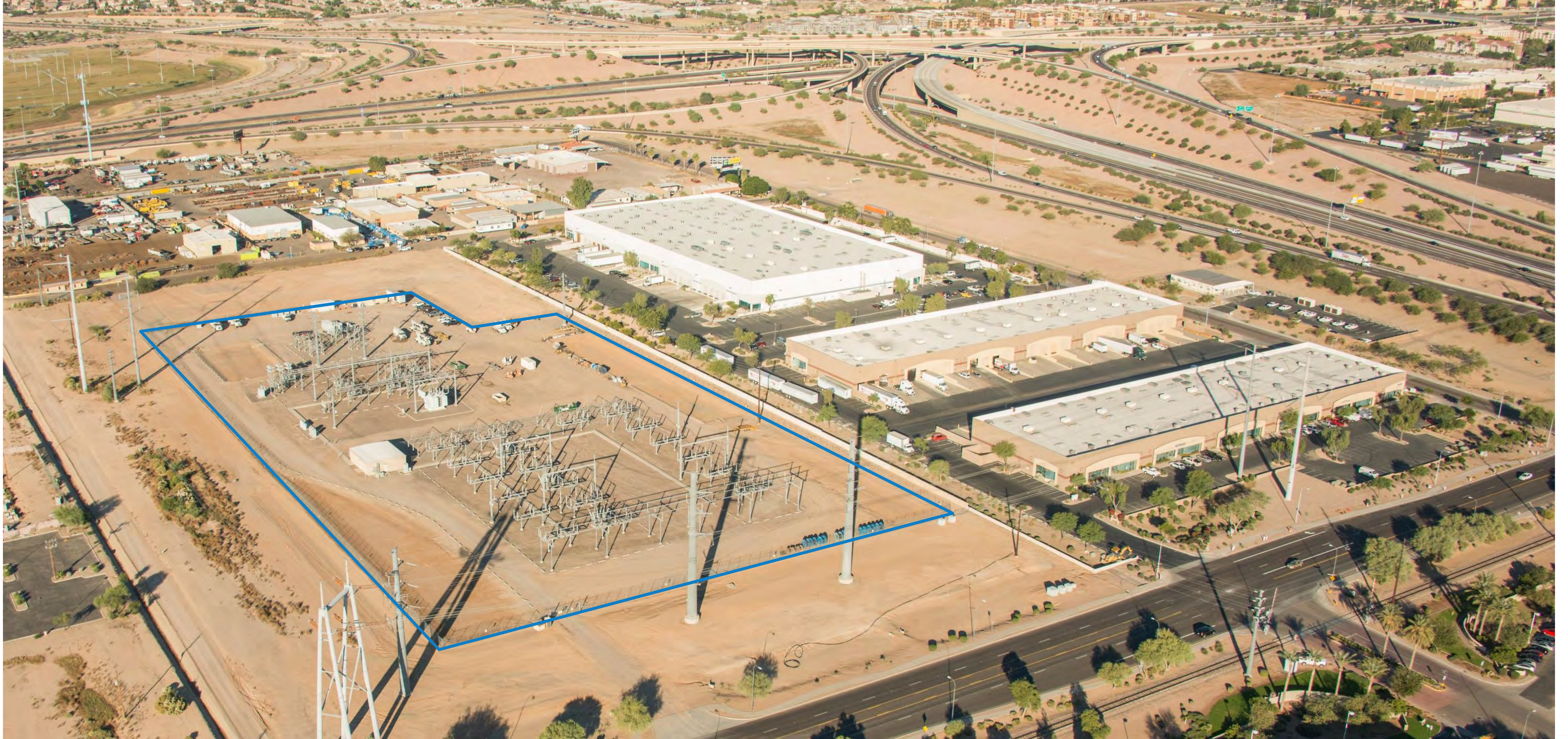
Typical 230kV Substation
